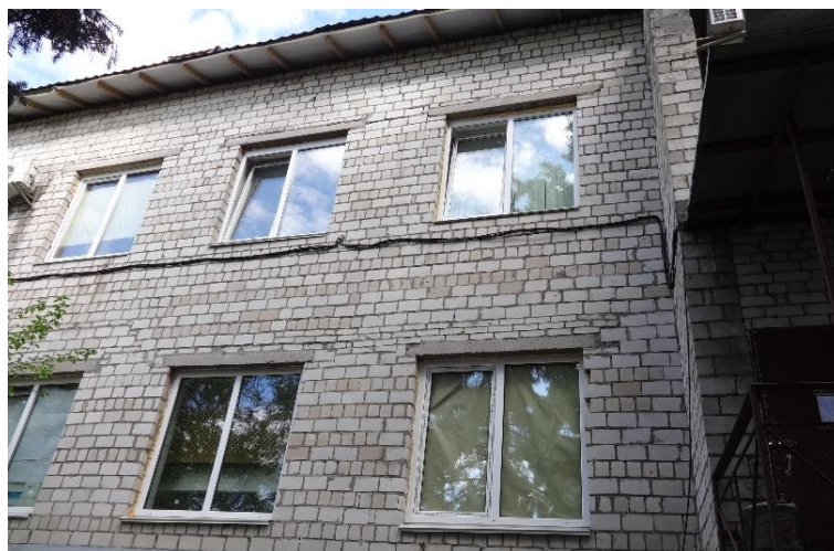
Fig. 2. Replacement of metal-plastic windows of the administrative building
